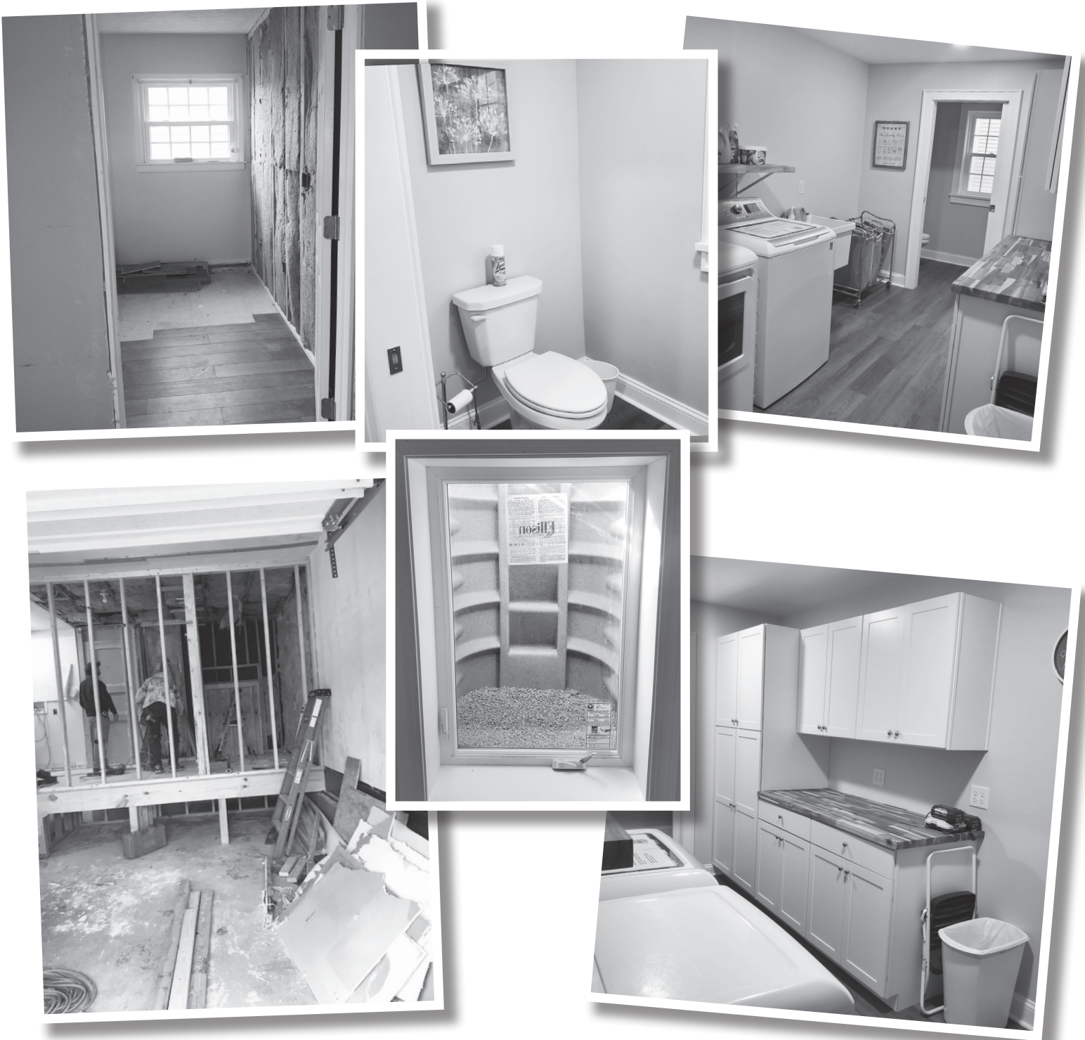
Expanded Laundry Room, Half Bath & Fire Exit Remodel.
